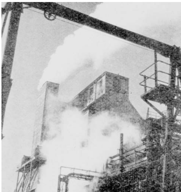
Figure 4 Coke oven plant in which bituminous coal is converted to coke for subsequent use in blast furnaces as an integral part of manufacture of steel. Workers assigned to “topside” positions closest to the top of the stack had highest rates of lung cancer (Hunter 1969)
